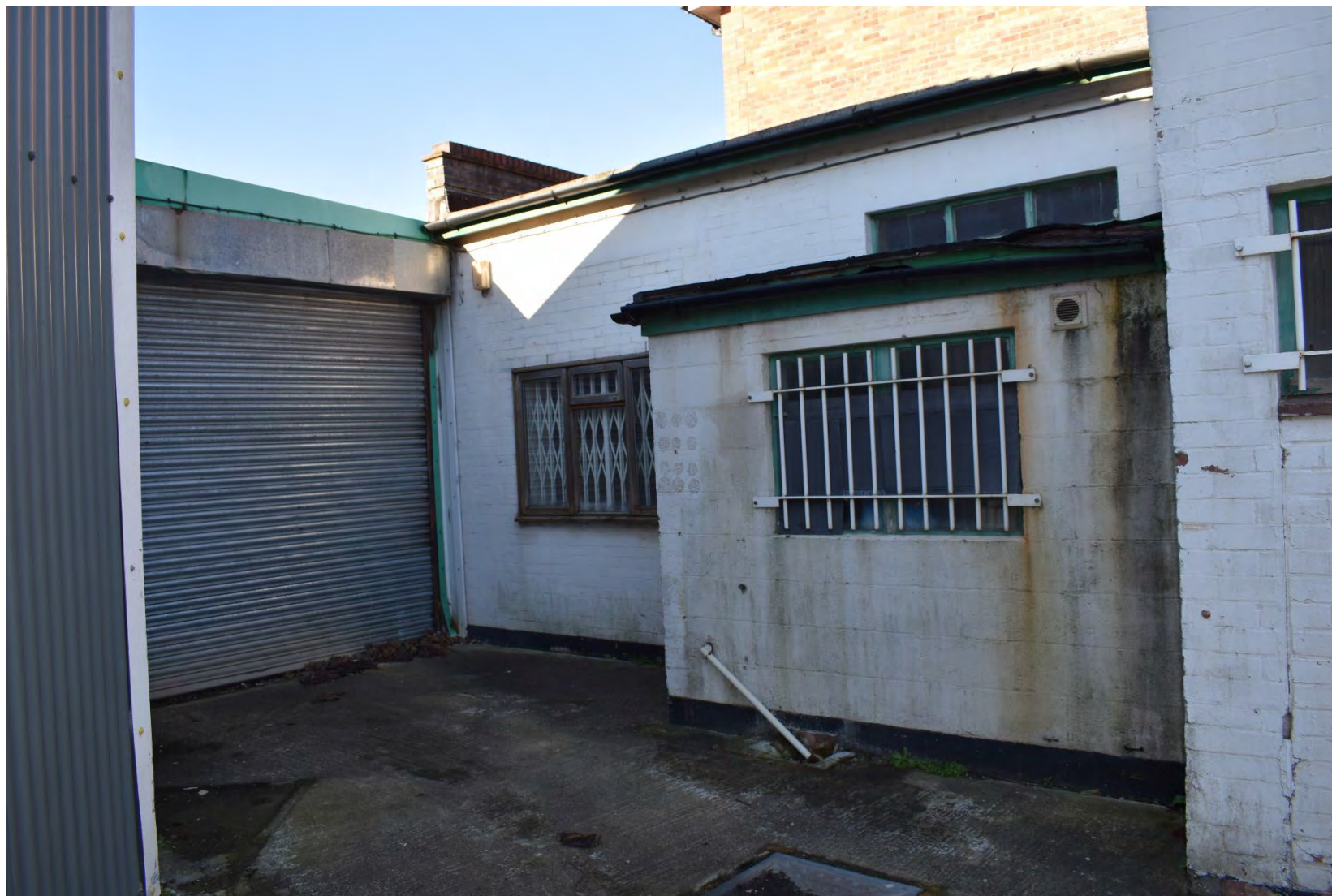
Plate 14: View of the buildings in the north western corner (facing NW)
