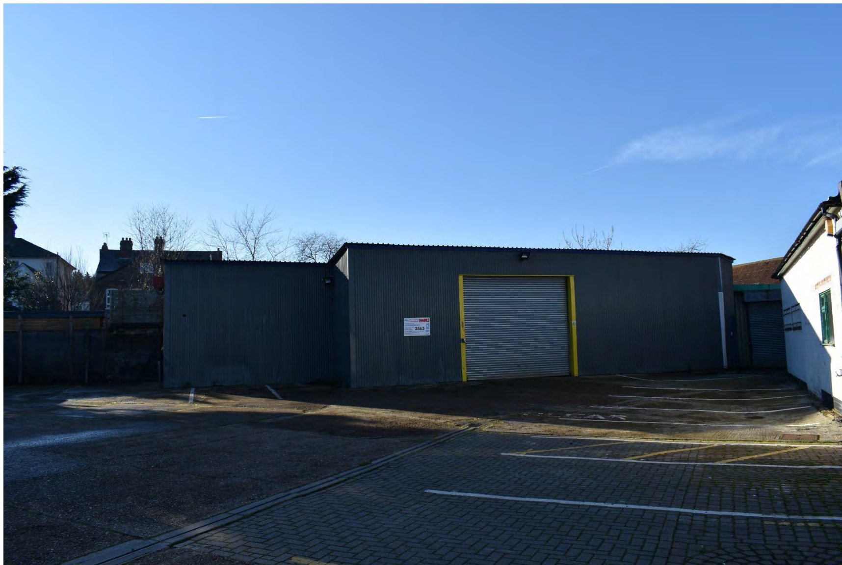
Plate 12: View towards the building on the western boundary (facing SW)
